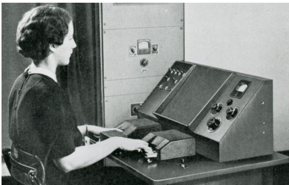
Figure 1.1: Image of mechanical vocoder the Voder by Homer W. Dudley [5].
